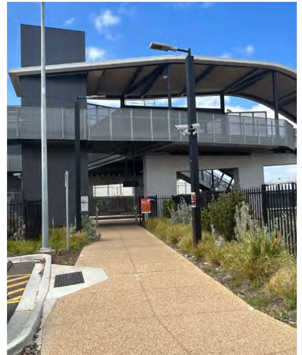
Figure 30 – Cobblebank Station entry and ramp
