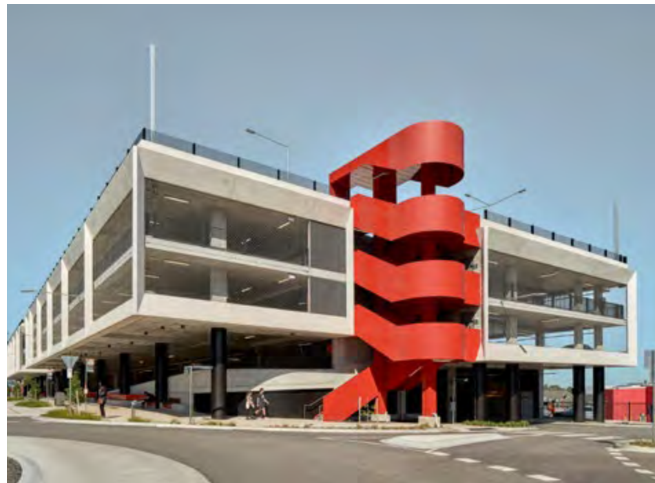
Figure 29 – Berwick Car Park and Bus Interchange. Source: Betterfutureawards
