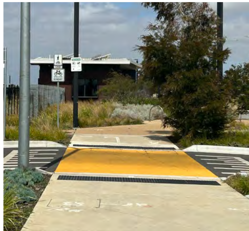
Figure 27 – Cobblebank Station Cycle Trail.
