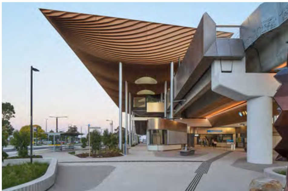
Figure 21 – Pakenham Station - Genton. Source: Genton
