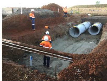
Figure 15. Upstream buried Culverts during construction
