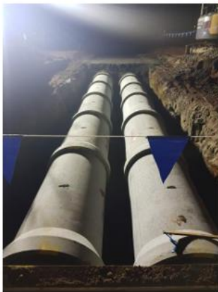
Figure 14. Upstream buried Culverts during construction
