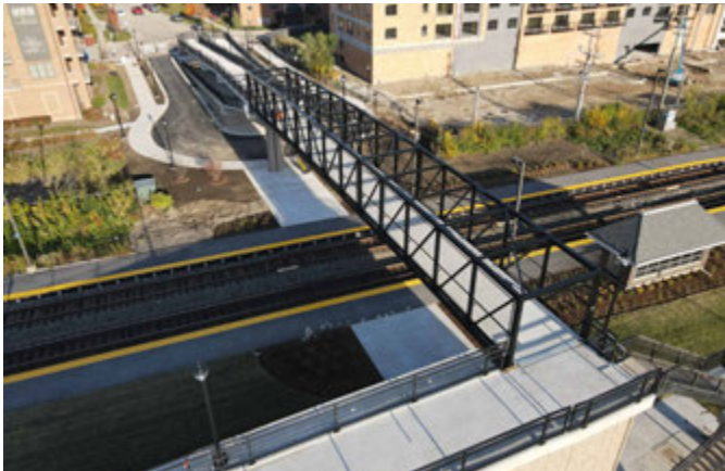
Figure 28 - Railway overpass in Mundelein, Illinois, HR Green
