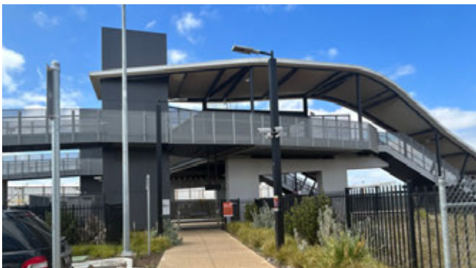
Figure 29- Railway overpass in Cobblebank, Victoria
