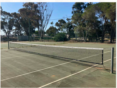
Public tennis court and netball court including seating and shelter in poor condition.
