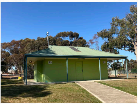
Public access toilet block in poor condition.
