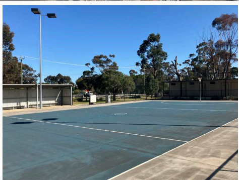
Multi-use court in good condition with portable change rooms and toilets.
