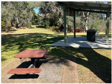
Picnic area at the Old Melton Reservoir in fair condition however lacking accessible path to amenities.
