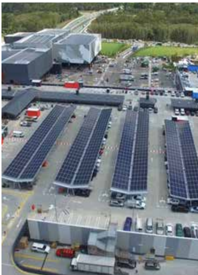
Solar car shade structures
